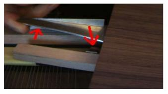
Pull up the enlongated piece of metal and pull the wood panel straight out towards you. You will notice a small red wheel attached to the panel that rolls underneath the metal. This is the damper mechanism.
